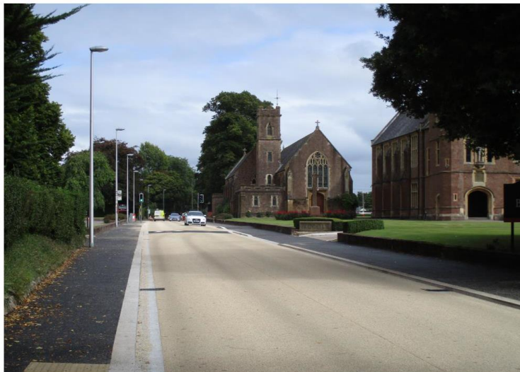
Completed Blundell's Road traffic calming improvements – October 2016
