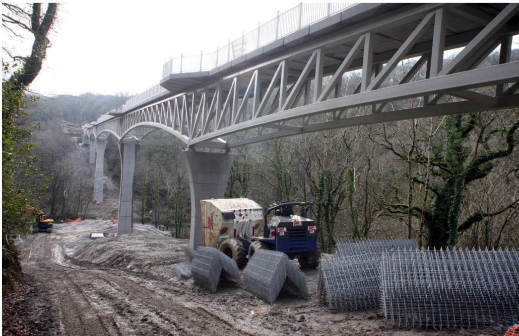
Gem Bridge (near Tavistock) Pedestrian / Cycleway 2013
